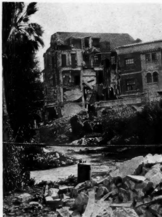
FIG. 3. SHOWING DEMOLISHED TOWER OF ARLINGTON HOTEL
